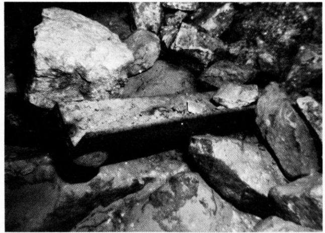
Plate rail found in the flooded slope shaft at Merstham. This rail is very similar to Type 1 rails, as observed in the Godstone quarries. Photo: the late John Maneely
